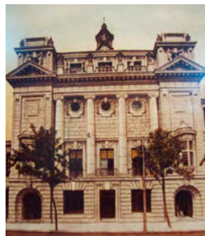
Shanghai Masonic Hall No. 30 The Bund 1865
